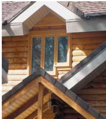
Enclose eaves and soffits.
